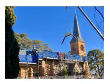
In 1960 asbestos tiles replaced the seriously deteriorated timber shingles on the St John's roof. From July to October 2019 these asbestos tiles were replaced with Welsh slate costing nearly \$400,000.
